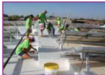
Mudslingers on the roof
